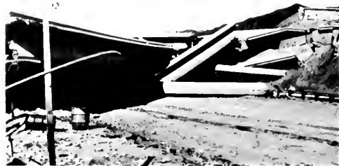
Photo 11. Damaged overcrossing at the Golden State Freeway and Foothill Freeway interchange [4].
